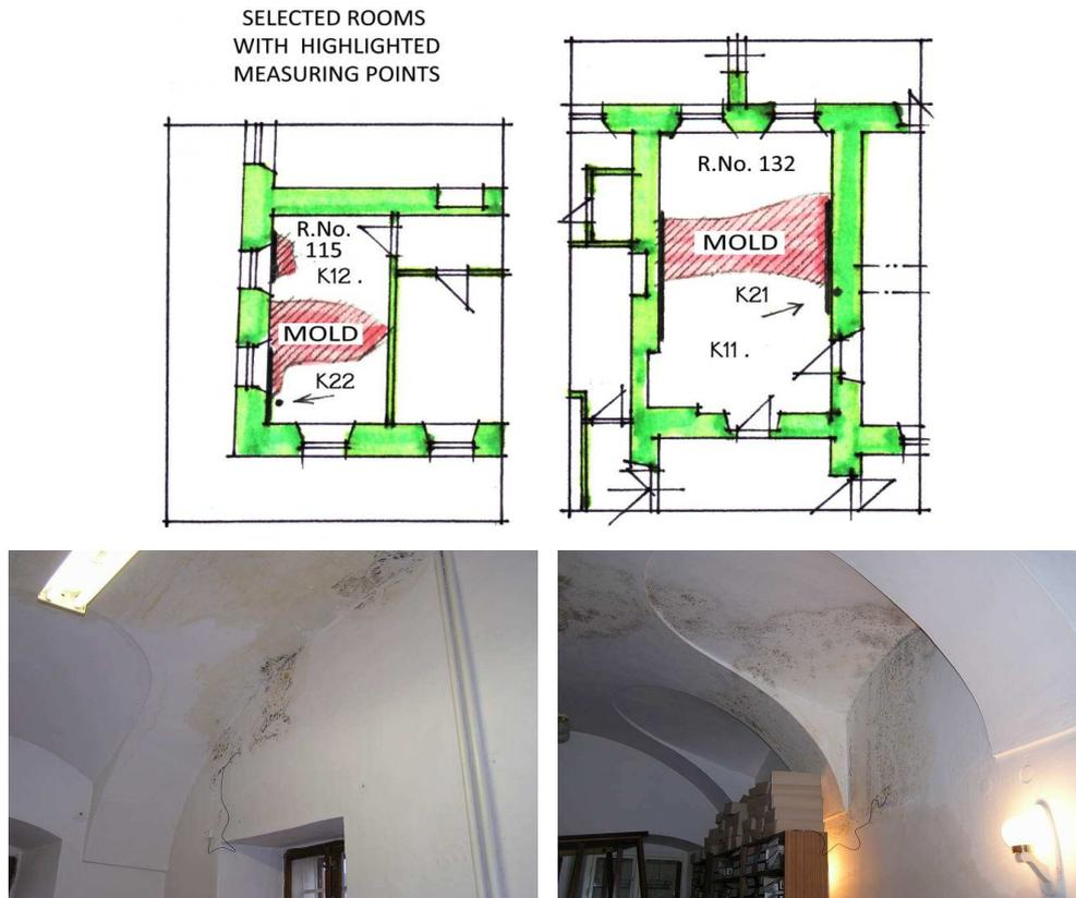
Fig. 2. Views of mildew occurrence in rooms No. 115 and 132 with positioned sensors
