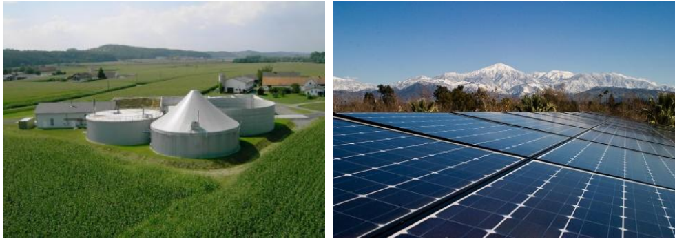
Fig. 1. A biogas plant (left) and a photovoltaic power plant (right)
