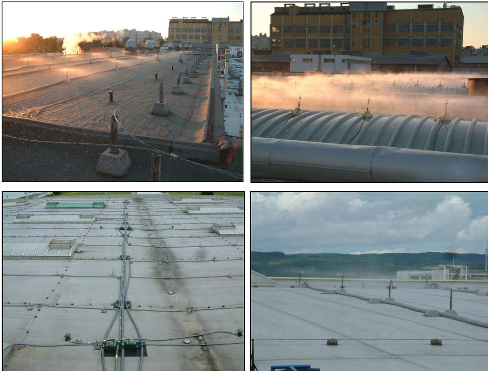
Fig. 1. Evaporative roof cooling system
