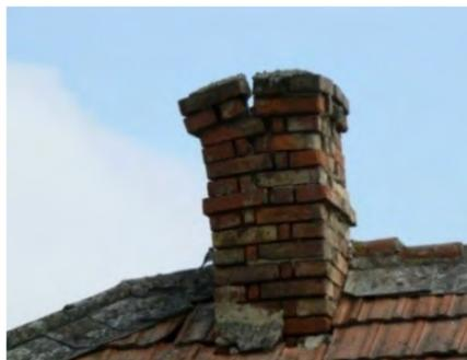
Fig. 13. Destruction of chimney body [source: the Internet]
