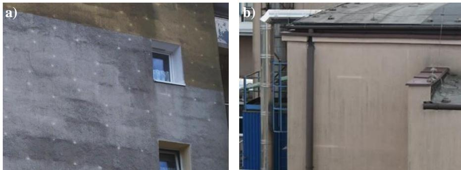
**Fig. 4.** Permanently soiled facades with acrylic plaster. Unsoiled surfaces in the area of: a) mounting pins, b) gaps between the panes (*own photos*)
