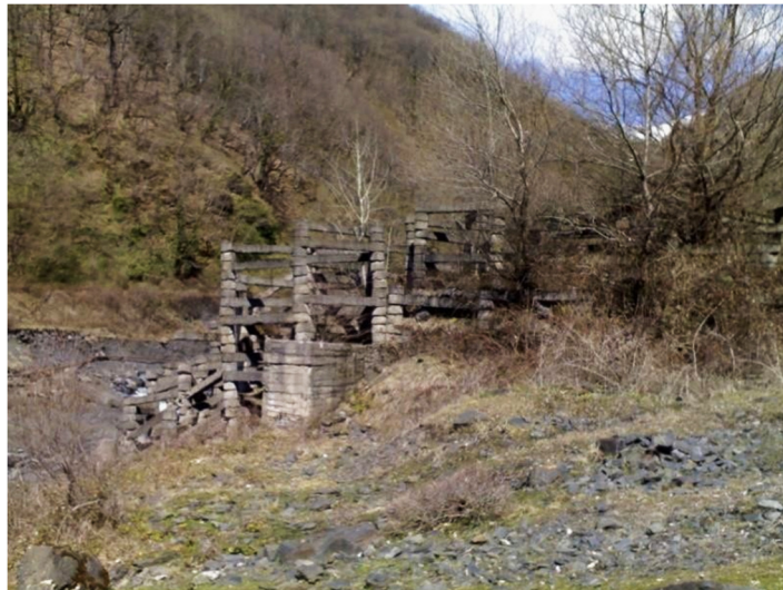
Fig. 1. I. Kherkheulidze's lattice-type mudflow-catching structure ( own photo )
