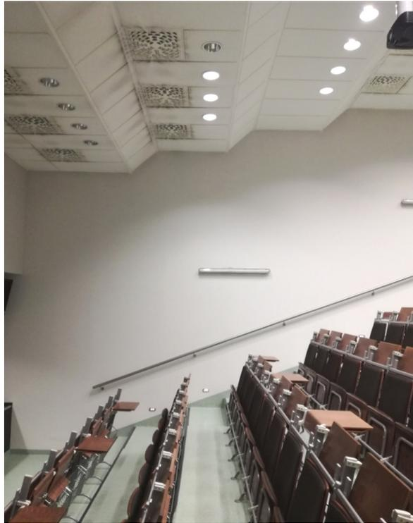
**Fig. 3.** All lamps in the first row and two middle lamps in the second row switched off in the case of lighting activated by controller during multimedia presentation (*own photo*)
